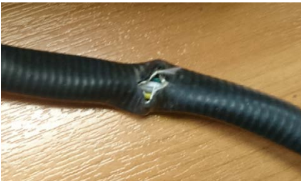
Figure 13. Damaged wire protector.
